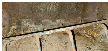
Steel elevated wood holder, allows wood to combust properly and burn completely.
