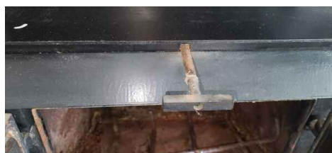
Damper control handle - pull to open and push to close the damper.
