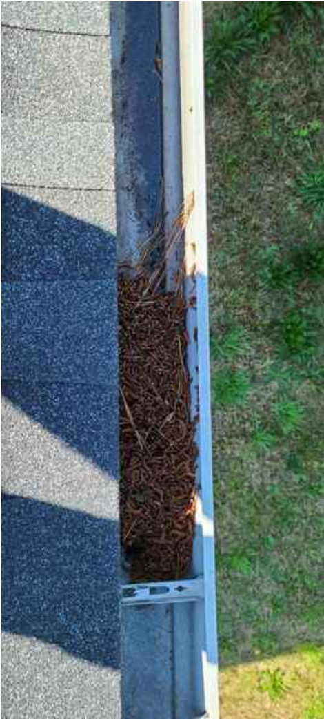
Debris in gutter needs to be monitored and cleaned regularly to prevent drainage problems.
