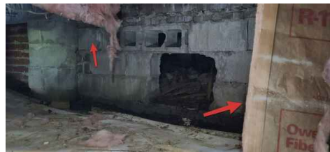
Falling insulation near front steps
