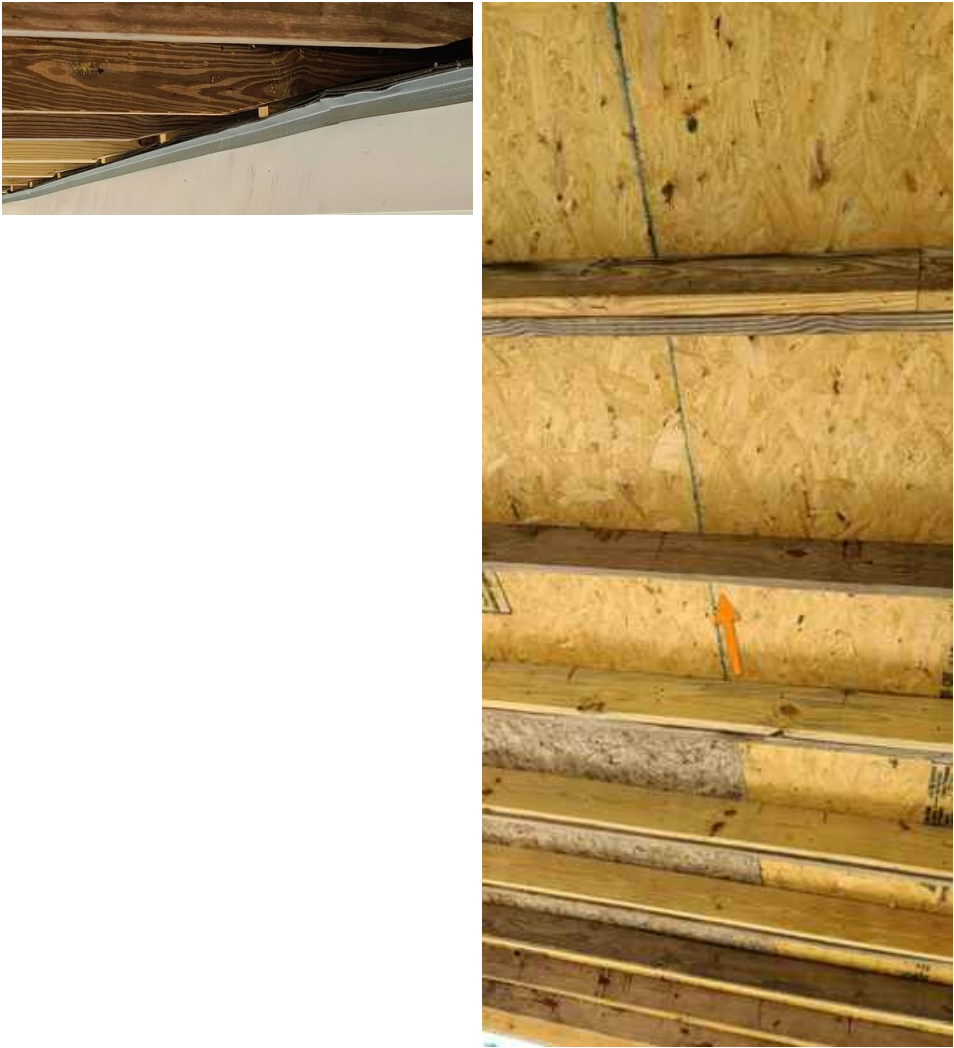
Rafter is not doubled—missing rafter.
